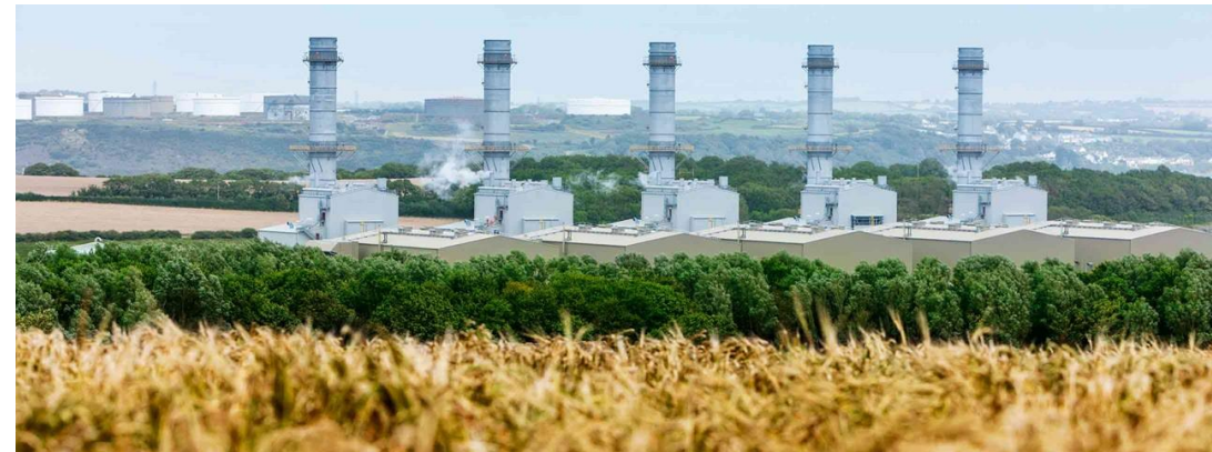
RWE Pembroke B gas fired power station
