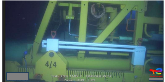
FIGURE 14: WMS AFTER INSTALLATION
