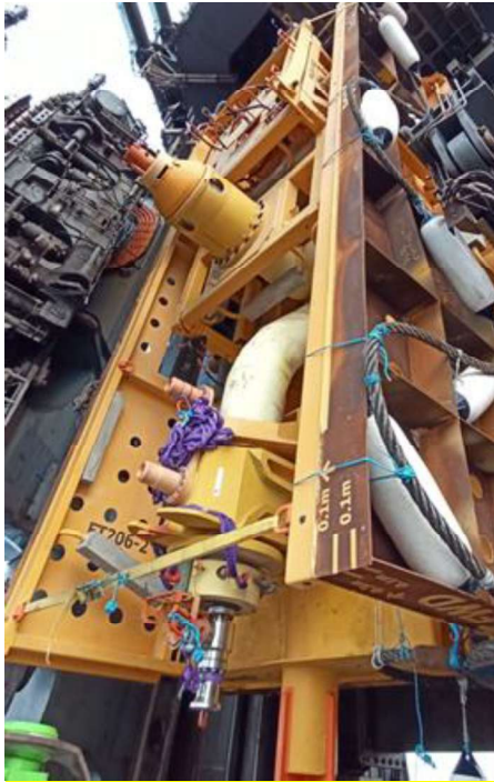
FIGURE 11: FIRST END FLET WITH WMS DURING TIE-IN OPERATION IN PIPELAY VESSEL
