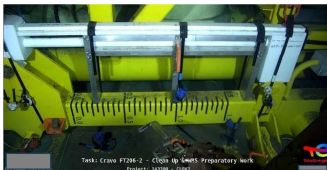
FIGURE 12: LATTICE WMS ON SEABED WITH LASHINGS
