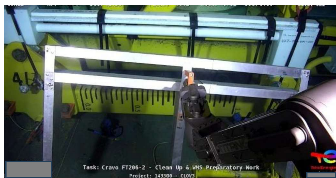
FIGURE 13: REMOVAL OF ALUMINIUM FRAME BY ROV
